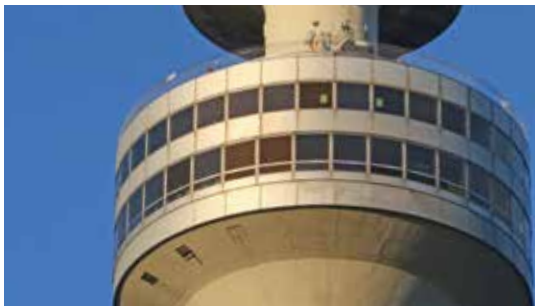
Restaurant 181 (Olympic Tower):
